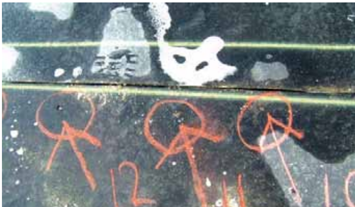
Breaches in Hot Rubber Membrane
