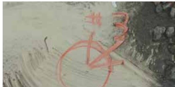
Breach in PVC Membrane
